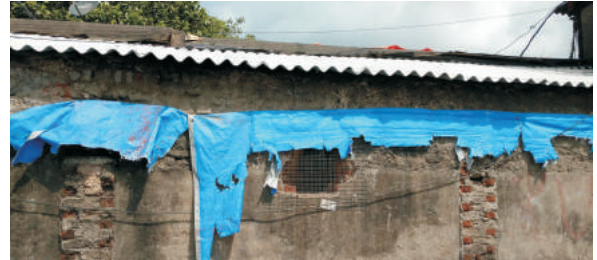
Roof repaired and set to begin with new admissions.
